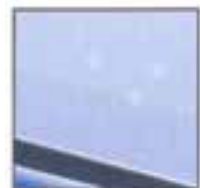
Multiple dents in a localised area.
