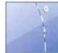
Excessive chipping of door edge or surround.
